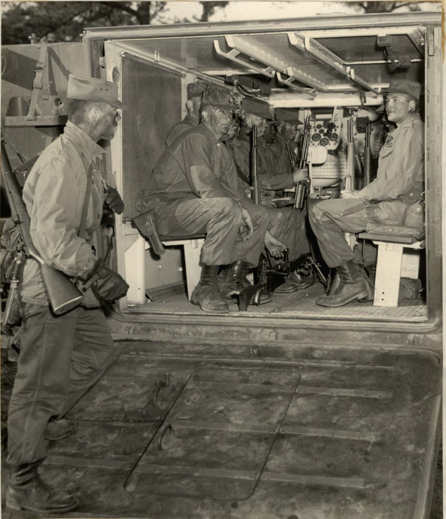
ANNEX C - TROOP COMPARTMENT, M-59 ARMORED PERSONNEL CARRIER.
